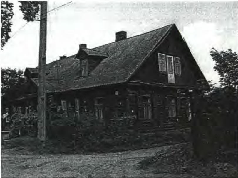
Image 2. Wooden house in Šnipiškės.
